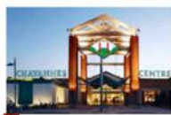
18 Chavannes Centre, Chavannes-de-Bogis (VD)
