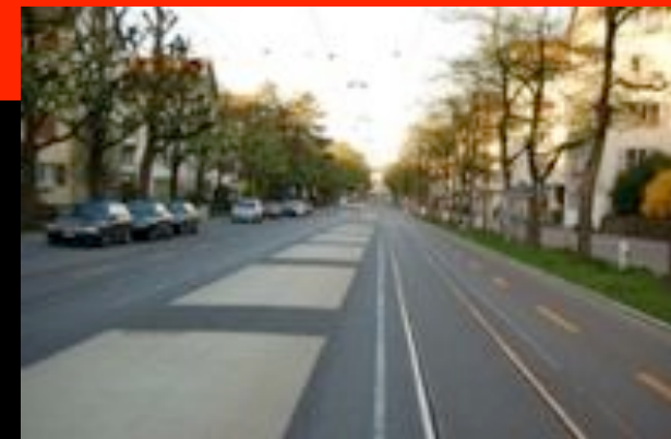
Tram Bern West
